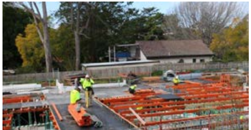
Then the foundations
